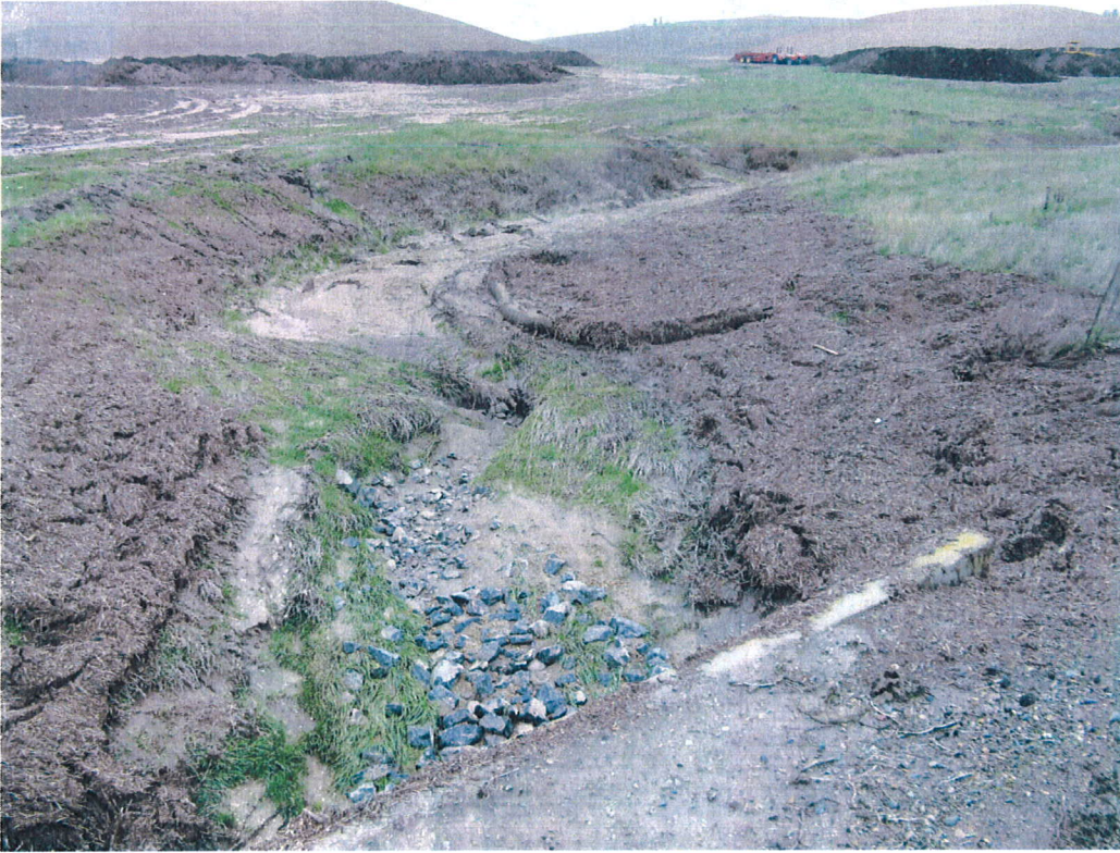
11Jan2008 - Lake Road looking SW at graded watershed runoff channel showing displaced wattle and manure piles; flow had backed up at culvert
