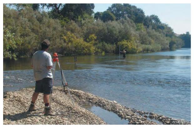
*Figure 9. Checking riffle crest elevations at Patch 1 prior to completing in-channel construction (Photograph courtesy of Friends of the Tuolumne).*
