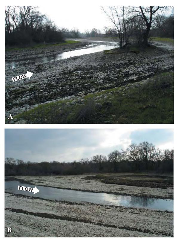
Figure 18. As-built high flow scour channel showing conveyance of flows from groundwater seepage during a dam release of 3,150 cfs. Photograph A) taken along the right side of the as-built floodplain at Station 16+00 looking downstream. Photograph B) Taken along the right side of the as-built floodplain at Station 16+50 looking back towards the main channel (Photograph courtesy of Friends of the Tuolumne).
