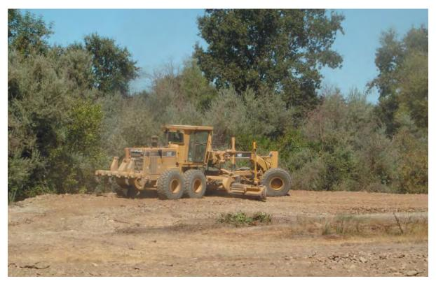
*Figure 3. Caterpillar 14H grader providing final grading elevations (Photograph courtesy of Friends of the Tuolumne).*
