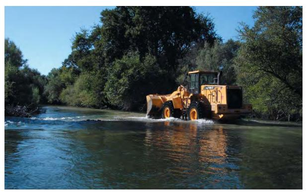
*Figure 8. Hyundai 770-7 front end loader placing and grading coarse sediment at Patch 3 (Photograph courtesy of Friends of the Tuolumne).*
