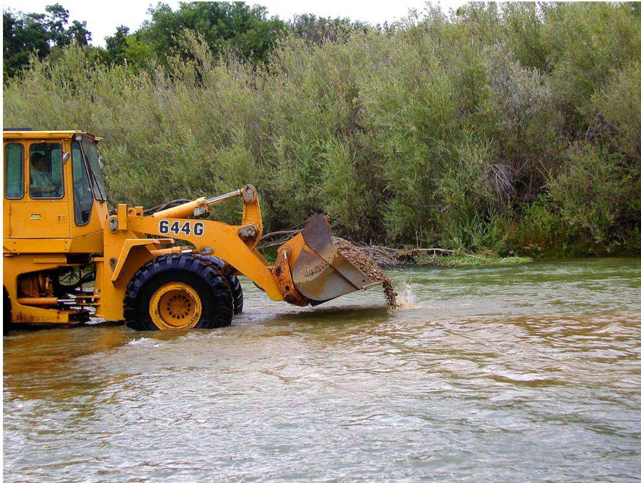
Picture 17 2003 – Riffle 15 b and 16, Front-end Loader Placing Gravel
