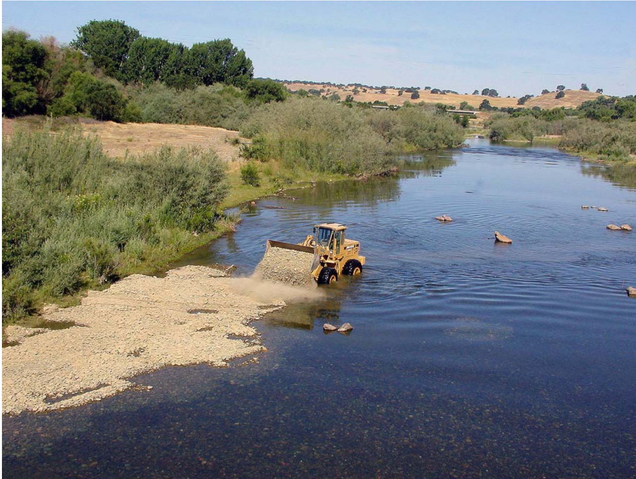
Picture 13 2002 – Riffle 15a, Slow, Flat Water as Construction Begins
