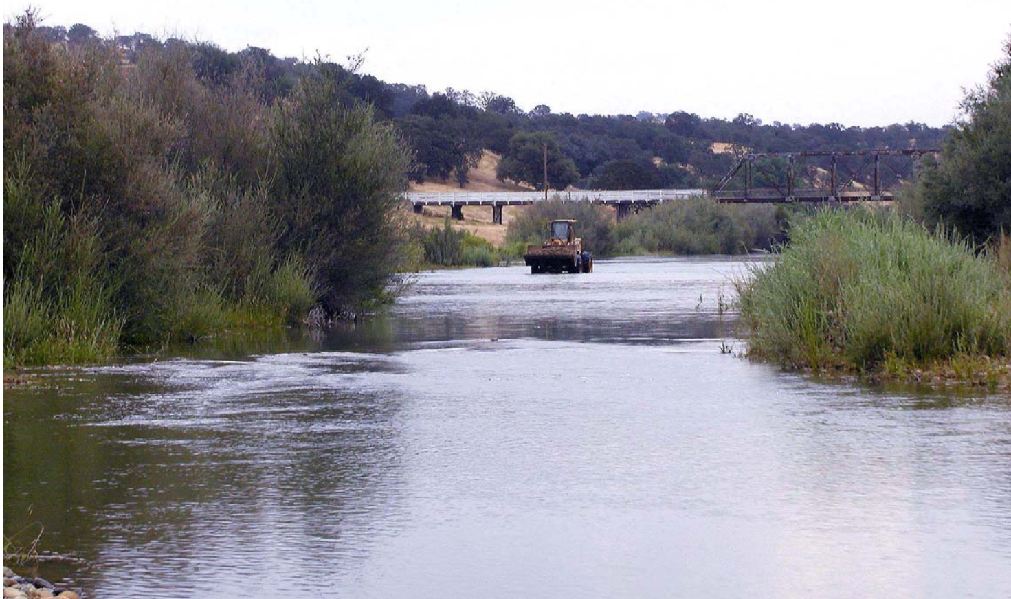
Picture 16 2003 – Riffles 15b and 16, Front-end Loader Carrying Gravel for Placement
