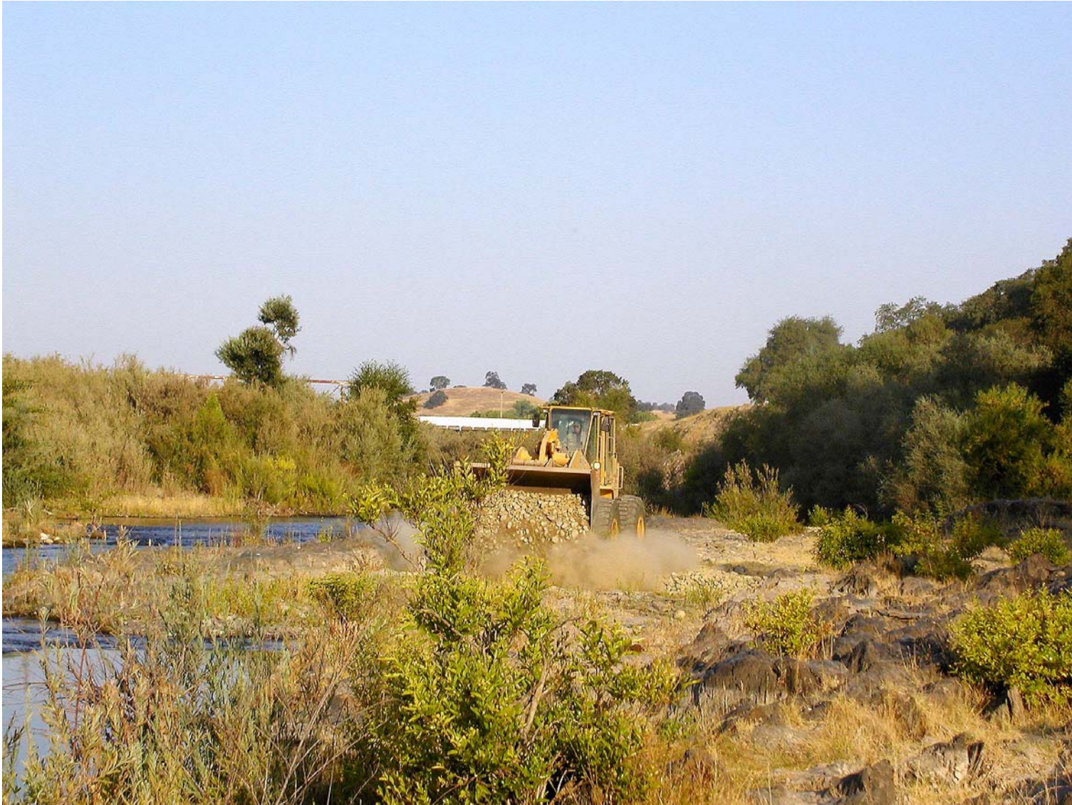
Picture 6 2002 – Riffle 12, Front-end Loader Places the Gravel
