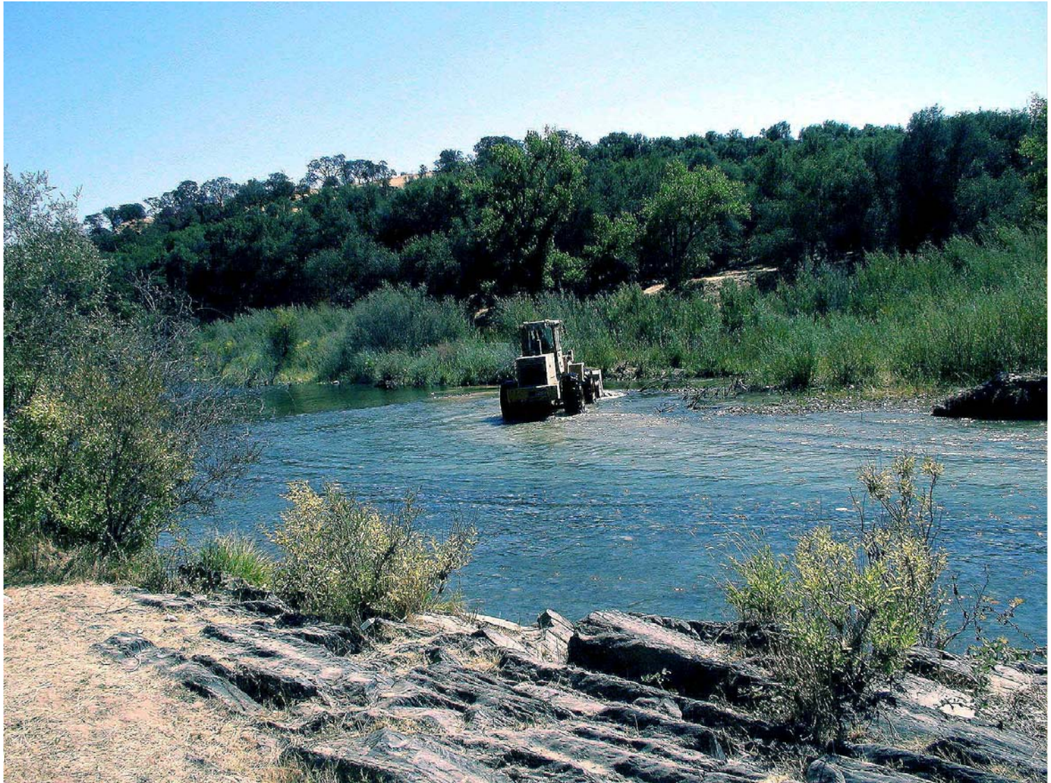
Picture 2 2002 – Building New Riffle 11
