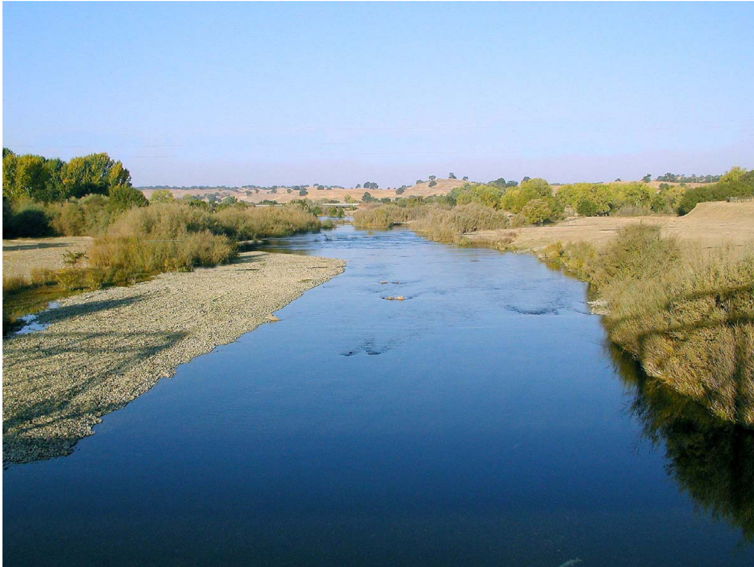
Picture 15 2002 – Riffle 15a Finished Creating a Source of Future Gravel and Narrowing the Channel
