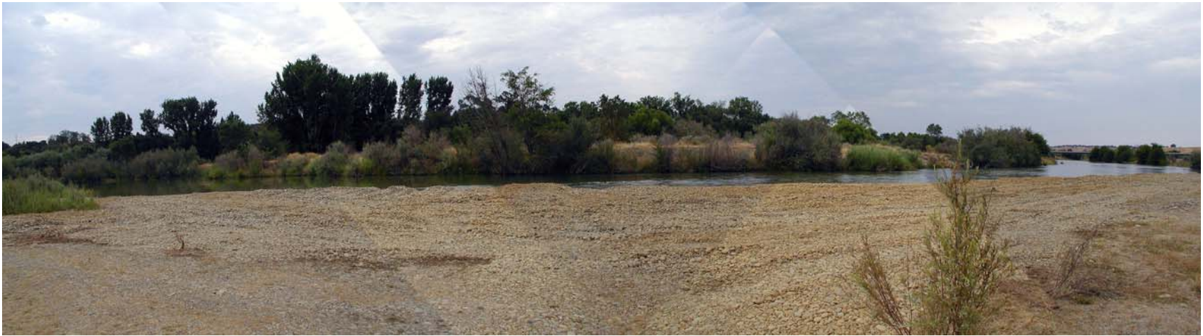
Picture 21 2003 – Riffle 18a and 18 b, Gravel Bar Created, Narrowing the Channel and Stockpiling a Source of Gravel to Migrate Downstream
