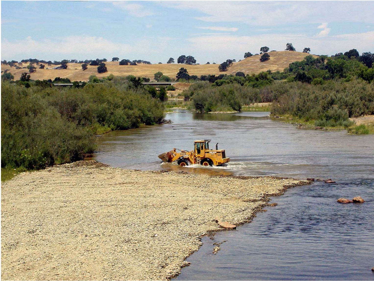
Picture 14 2002 – Riffle 15a, Front-end Loader Building Riffle
