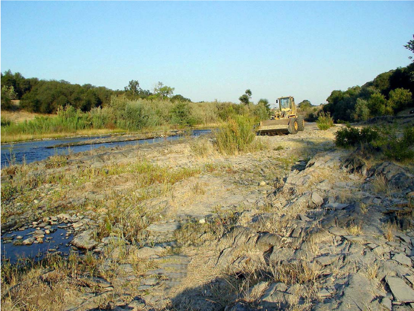
Picture 4 2002 – Riffle 12 is Bedrock Prior to Placing Gravel
