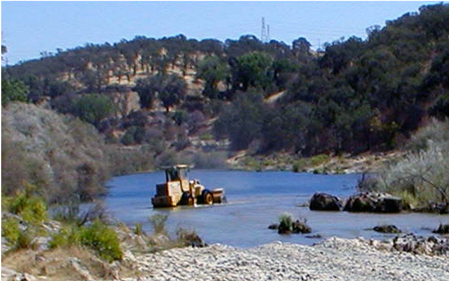
Picture 1 2002 – Building New Riffles by Extending Riffle 13 and Creating Riffle 11
