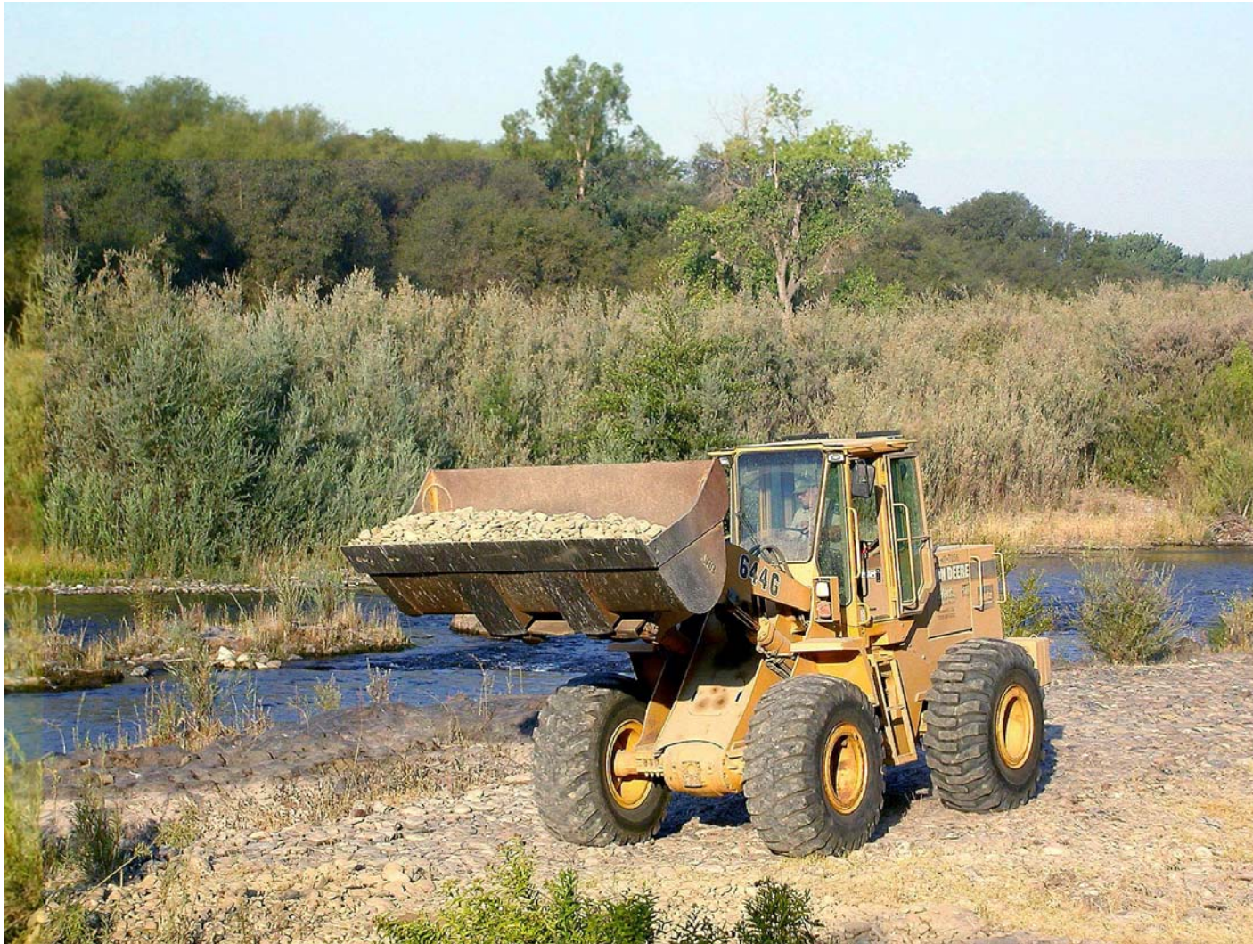
Picture 5 2002 – Riffle 12, Front-end Loader is Ready to Place the Gravel
